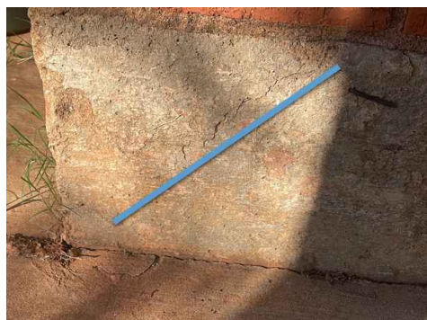
South West Wall
