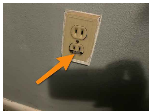
East Wall Primary Bedroom
