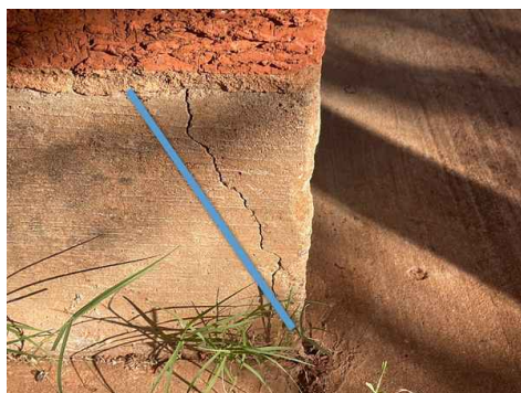
South West Wall
